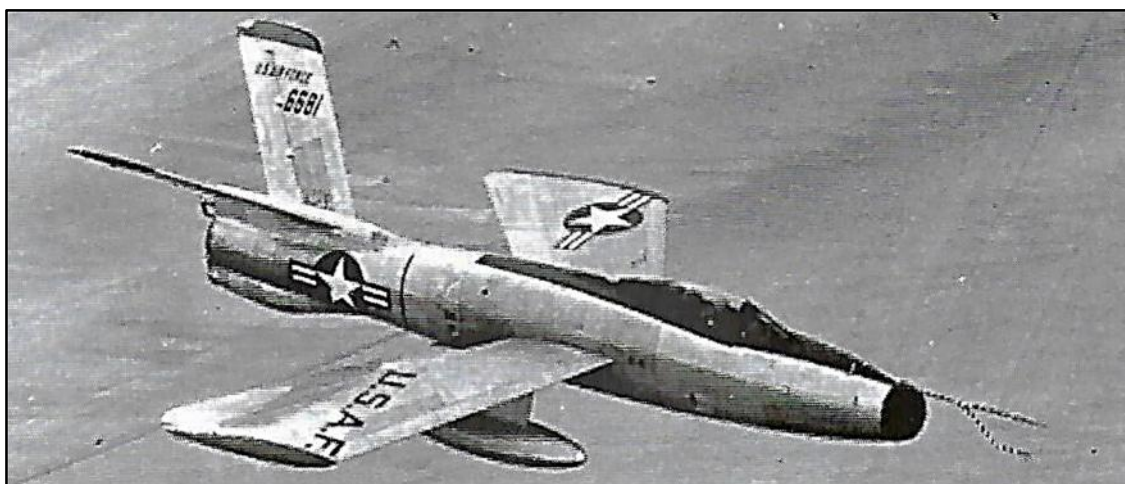
The second prototype as originally designed with 'V' tail
